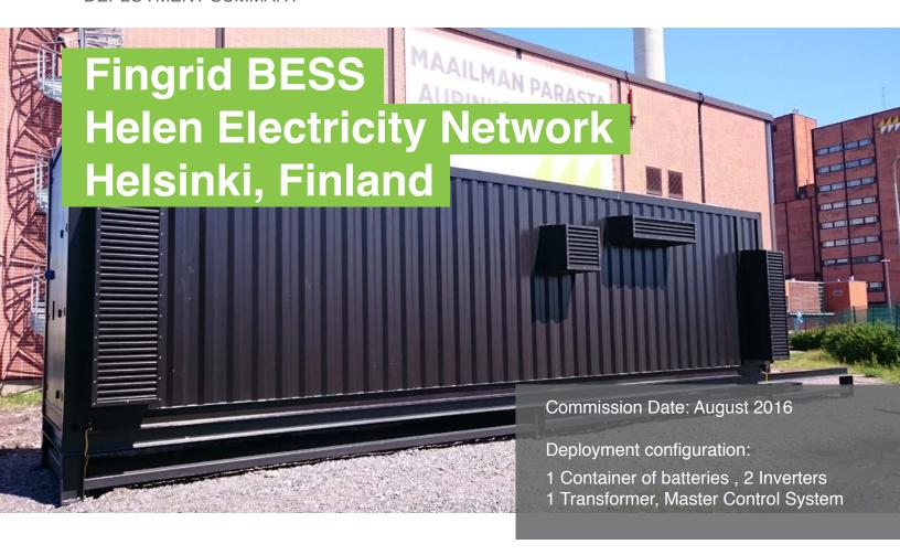
A turnkey AC battery storage system with 4-year service agreement is helping Helen Electricity Network and Fingrid to optimally dispatch PV energy to the grid on a daily basis.
