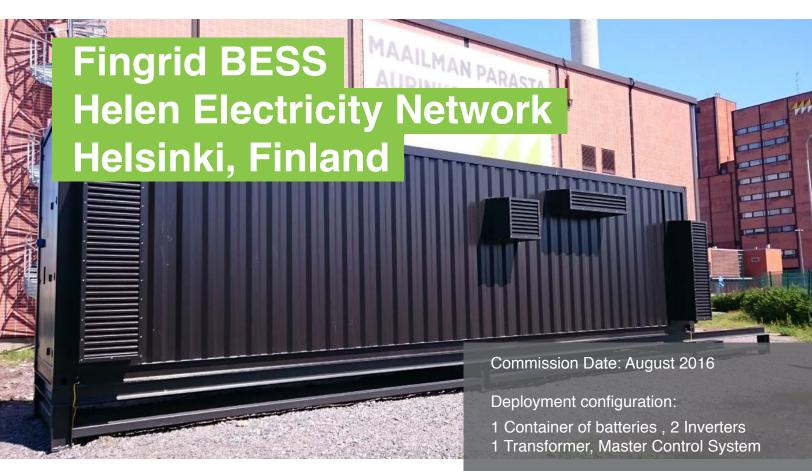
A turnkey AC battery storage system with 4-year service agreement is helping Helen Electricity Network and Fingrid to optimally dispatch PV energy to the grid on a daily basis.
