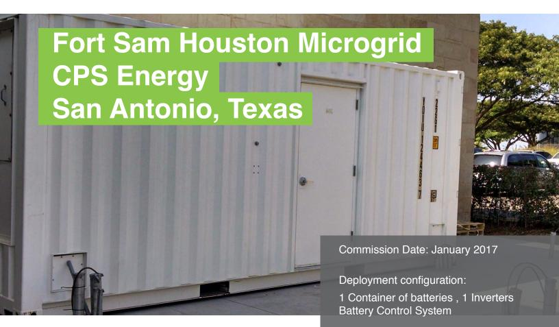
A turnkey AC battery storage system with 5-year performance warranty. The storage system is integrated into a utility-owned microgrid for testing the interoperability of multiple technologies at Fort Sam Houston.
